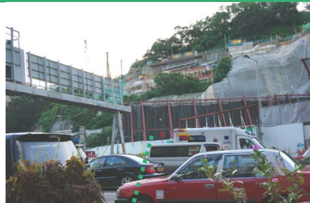
Vinyl Barrier mats are affixed on the metal framing at recent Railway Tunnel construction project, Hunghom, KTE1001
